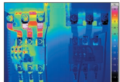
Inspection of electrical installations
