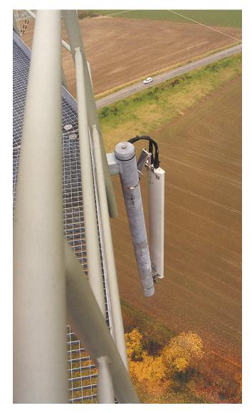
Photo 15: Installation of antennas: Upside-down. Cable is led directly upwards to the platform.
