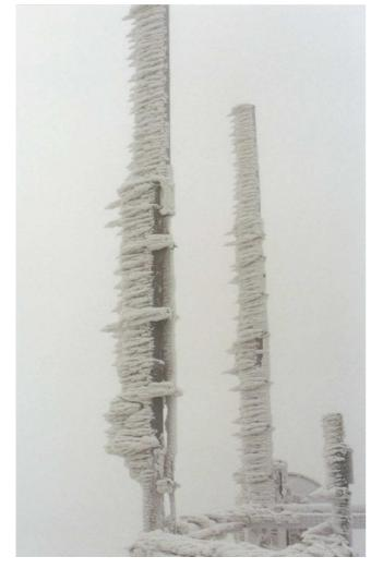
Photo 3: Iced up Kathrein omni-directional antennas – fully functional!
