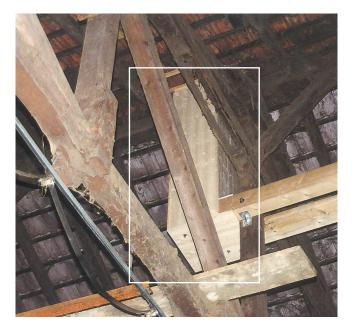
Photo 23: Disguised antenna mast in a shed barn.
