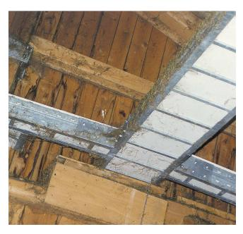
Photo 24: Fire protection of a cable path rinne in a shed barn, in accordance with fire protection class F90.
