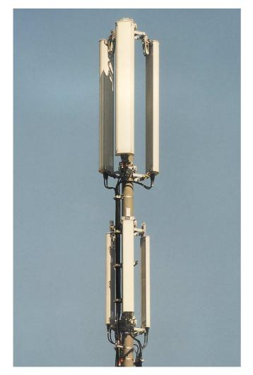
Photo 12: Cable led upwards behind antennas mounted at a distance.
