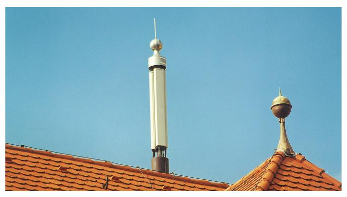
Photo 22: Antenna configuration adapted to suit the surroundings
