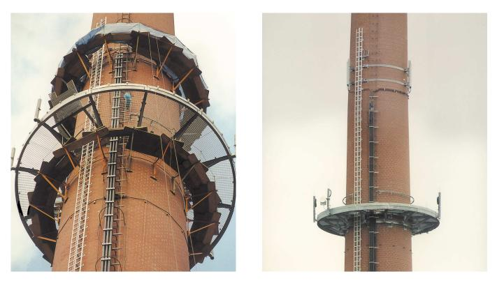
Photos 10 and 11: Installation of an antenna platform at a height of approx. 50 m with the help of two auxiliary platforms.
