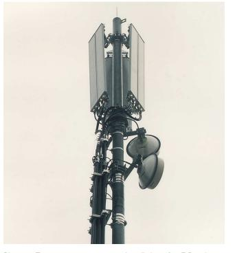
Photo 2: Two antennas per sector. Installation of 2 F-Panels per sector using 2 x F-Panel Mounting Kits.
